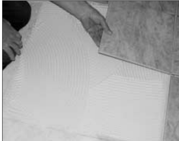
Figure 43: Thin set is combed with the notched side of the trowel.
