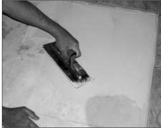
Figure 42: Thin set is “burned in” with the flat side of the trowel.
